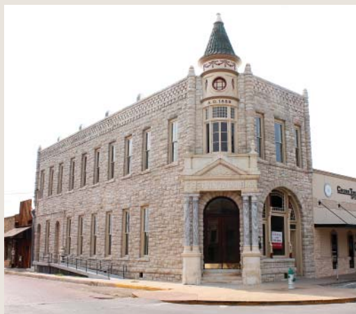
First National Bank, Stephenville, TX. Photos: NPS files
